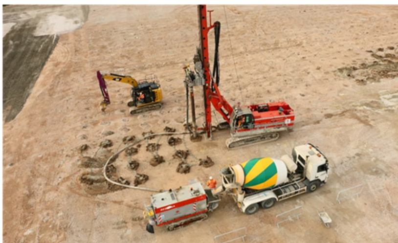
Figure 8 - CMC setup on site
